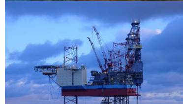
Drilling of geo-pilots ongoing
